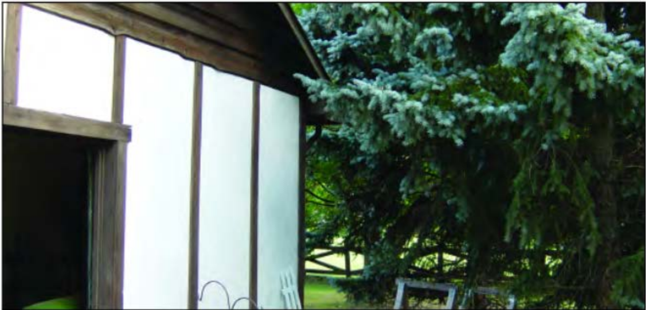
Figure 3 The spruce trees in this photo are located too close to the house. If they catch fire, they will likely create enough radiant heat to ignite the home. (Courtesy of MSU Extension.)
